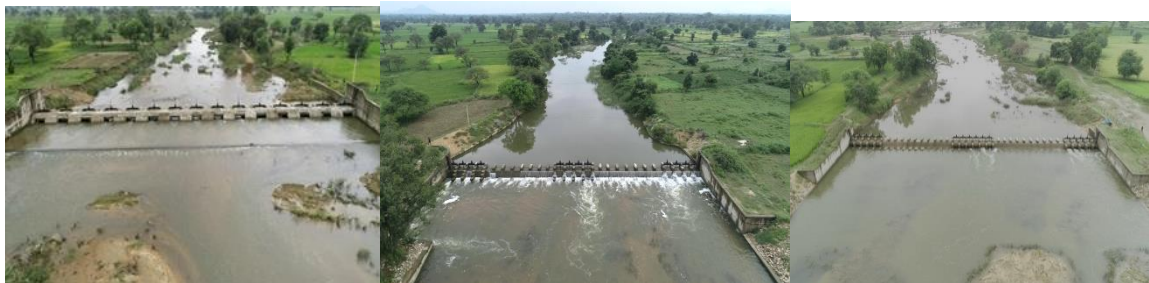
Figure 3 : CHECK DAMS AT BUDHIPALLI, PALSABHADAR AND PARKOD
