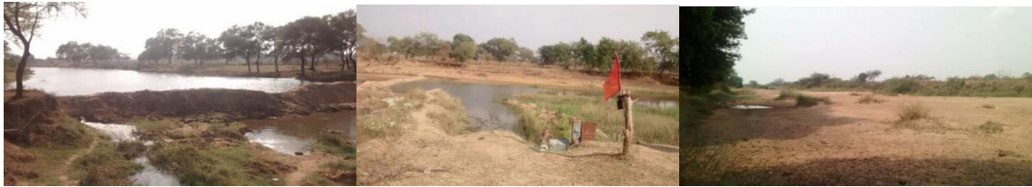
Figure 2:PRE CONSTRUCTION PHOTOS OF CHECK DAM AT BUDHIPALLI, PALSABHADAR AND PARKOD
